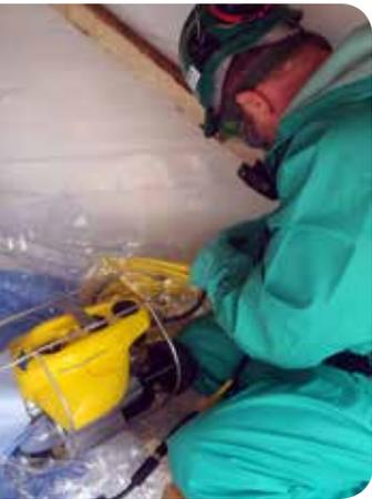
Preparing an ROV for water tank entry.
