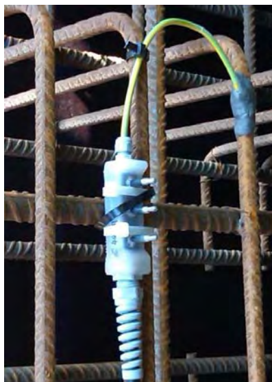
Figure 8 Modified M3 probes ready for casting into a reinforced concrete structure.
