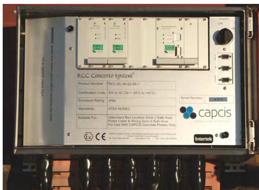
Figure 7 Rate of Corrosion in Concrete (RCC) Monitoring Instrumentation
