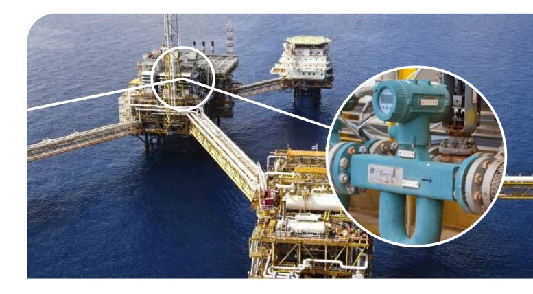
The use of Coriolis flow meters has become increasingly commonplace in the offshore oil and gas industry, as they are one of the most reliable instruments with which to determine flow measurement.
