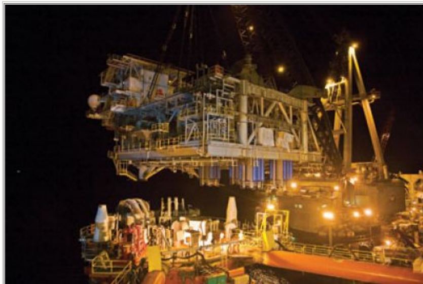
The utility module being installed at night. Photo by Coles Hairston.
