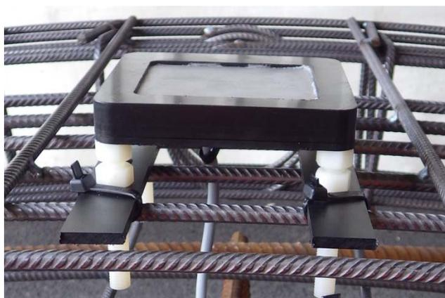
Figure 6 – Sense electrode installed onto rebar cage
