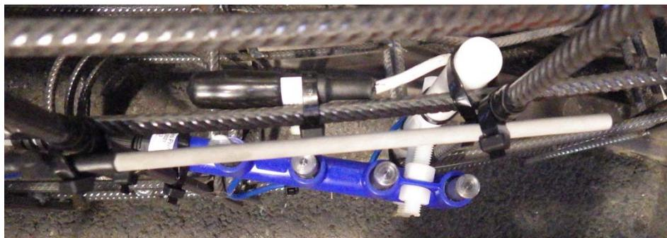
**Figure 3 – M4 probe installed into reinforcement cage**
