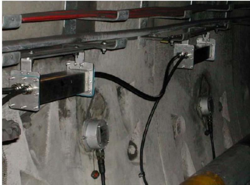
**Figure 17 – Instrument pods and installed C4 probes**
